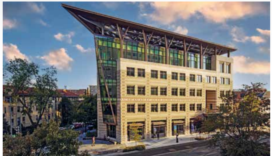
The American Geophysical Union Building (AGU).
