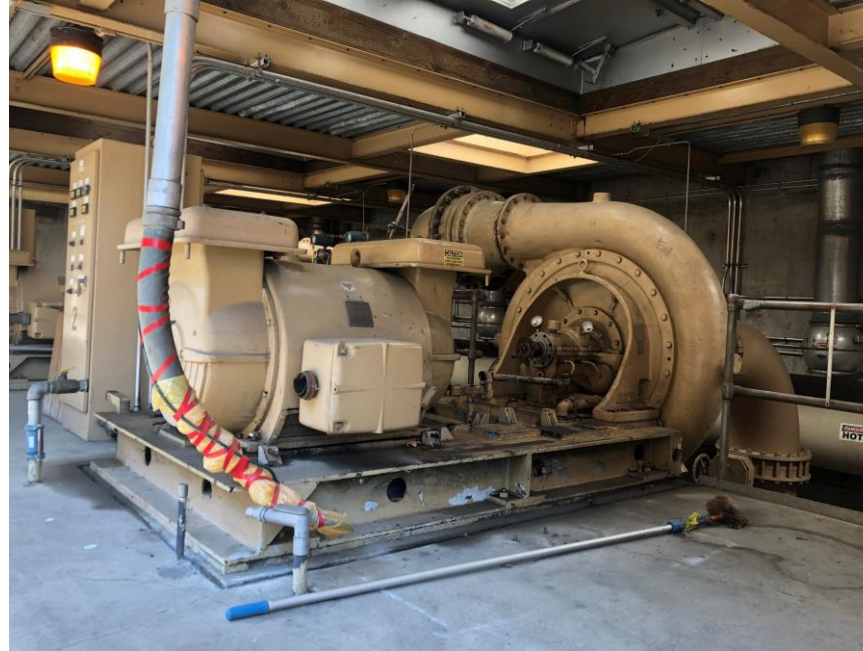
Original Blower Demolition
