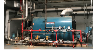
Digester Gas-fueled Boiler
