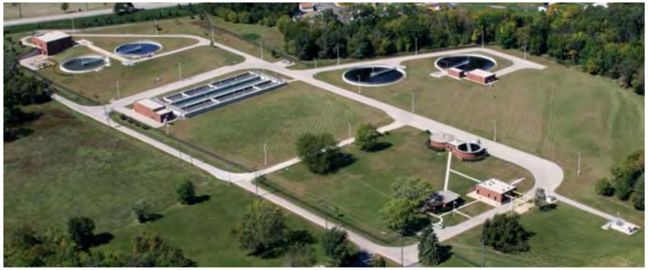
FRWRD's 5 mgd West Water Reclamation Facility – facilities were laid out for capacity expansion to 25 mgd.
