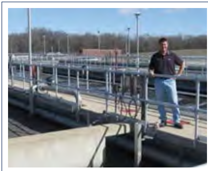
FRWRD's Superintendent Doug Haacker stands at the West plant aeration system, which is divided into five zones by concrete baffle walls.
