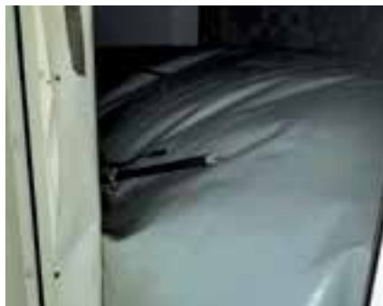
Gas storage bubble on the top floor of the brewery.
