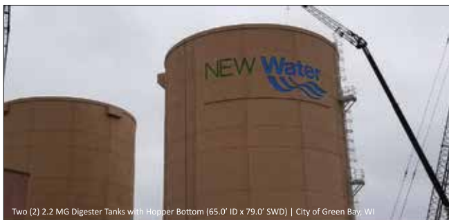
Two (2) 2.2 MG Digester Tanks with Hopper Bottom (65.0' ID x 79.0' SWD) | City of Green Bay, WI
