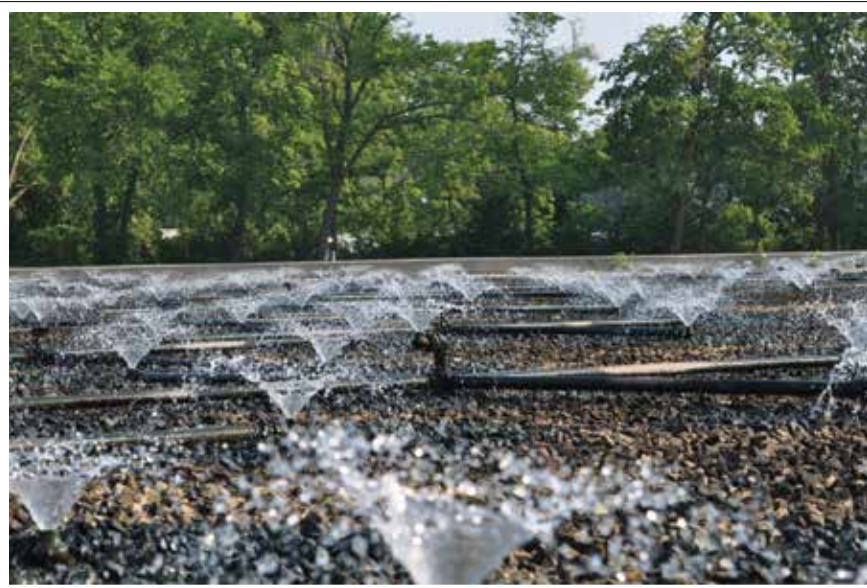
Trickling Filter at NEP: The 2016 image shows the flows just starting to increase.
