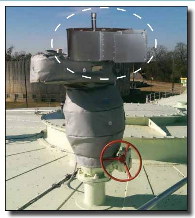
97570 with All-Weather Conservation Vent and Flame Arrester with Insulation Jackets
