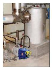
Sediment Trap with Electrically Actuated Drip Trap
