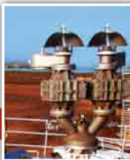
Dual 97571 with 97190 Safety Selector Valve on Digester
