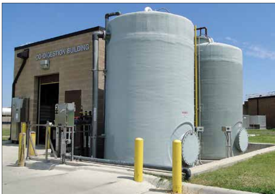
The co-digestion building is where the plant receives industrial wastes. Operators ensure that the wastes do not contain chemicals that would upset the anaerobic digestion process. (Credit: Kristina Twigg)
