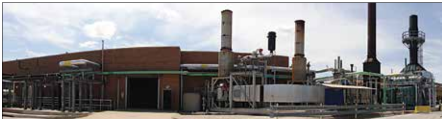
The Village Creek Water Reclamation Facility generates both energy and steam. The steam is used to power two of the plant's aeration basin blowers. (Credit: Kristina Twigg)
