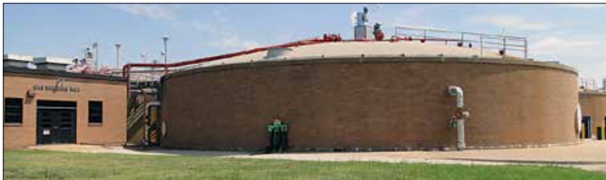
Biogas, used to generate energy via the plant's turbines, is created in these anaerobic digesters fitted with linear motion mixers. (Credit: Kristina Twigg)
