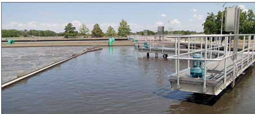
Using anoxic zones in the aeration basin improves energy efficiency at the Village Creek Water Reclamation Facility. (Credit: Kristina Twigg)
