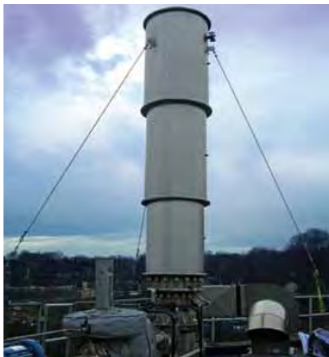
97311 Enclosed Waste Gas Burner with Ground Level Pilot Ignition
