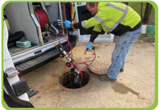
Operator Tim Hendrickson Cleaning Televising Camera
