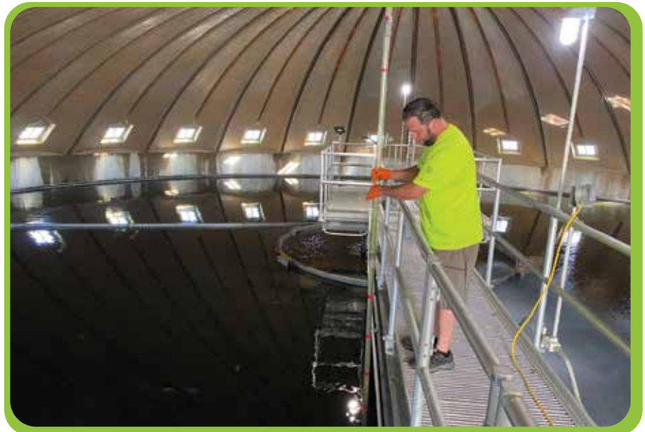
Operator Chris Molidor Measuring Sludge Blanket
