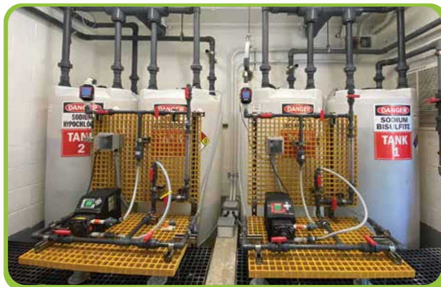
Disinfection Chemical Storage and Feed
