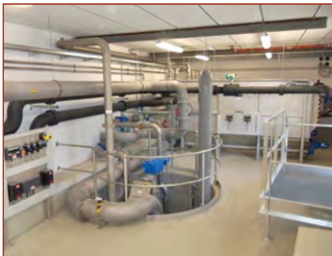
Figure 6: Central facility control room with wastewater shaft (RoK 4 in tank) and wastewater heat exchanger in the background.
