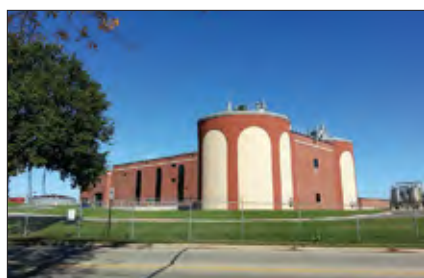
WAS Thickening and Acid Digestion Facilities constructed during the 11th Addition Project
