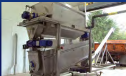
DSP Screw Press Model 3012, NY WWTP
