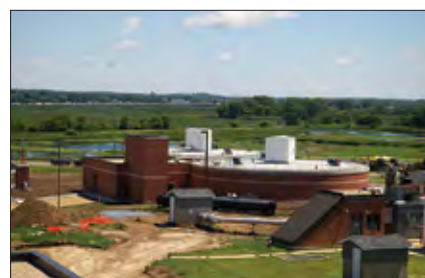
First Stage Thermophilic Methane Digesters
