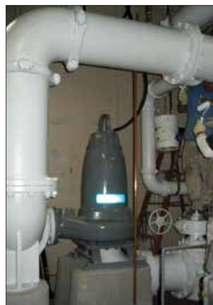
PHOTO 2: NEW VERTICAL-MOUNTED DRY-PIT SUBMERSIBLE PUMP
