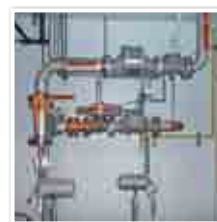
Pressure Regulator Flame Trap Assembly
