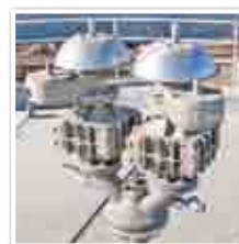
P/V Vent, Flame Arrester & Safety Selector Valve
