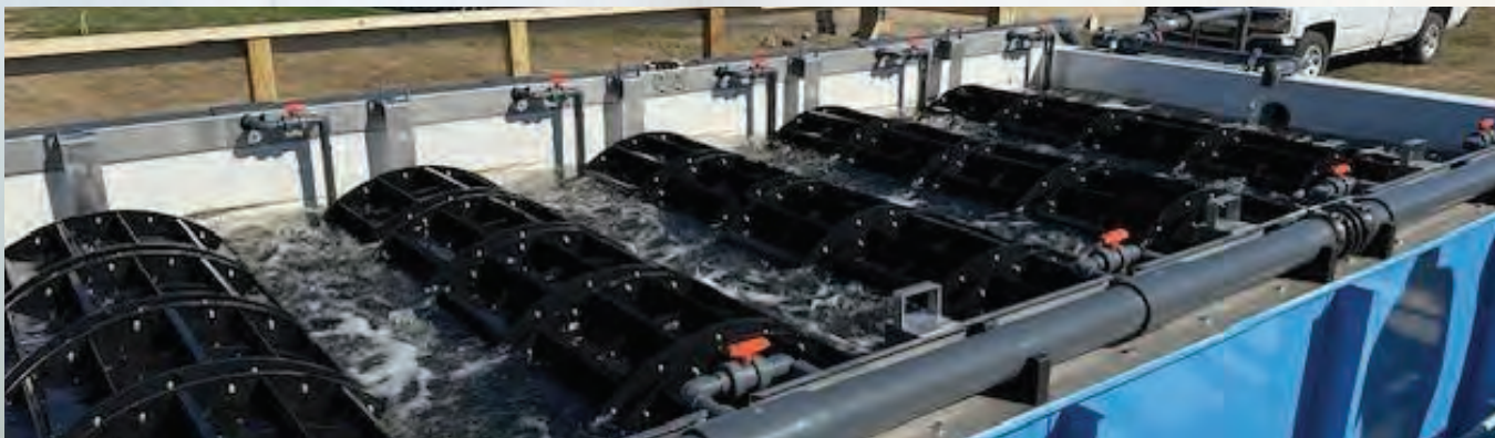
Image 3: FRWRD Algaewheel™ Pilot Reactor, October 2024.
