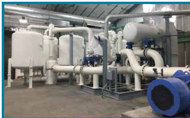
WLSSD's two vacuum swing adsorption units serve as the primary source of high-purity oxygen (90%+) gas.
