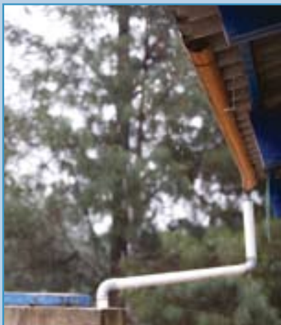
A natural solution: the rain flows down the roof, is captured in a gutter and flows through a pipe into a cistern near each house.
