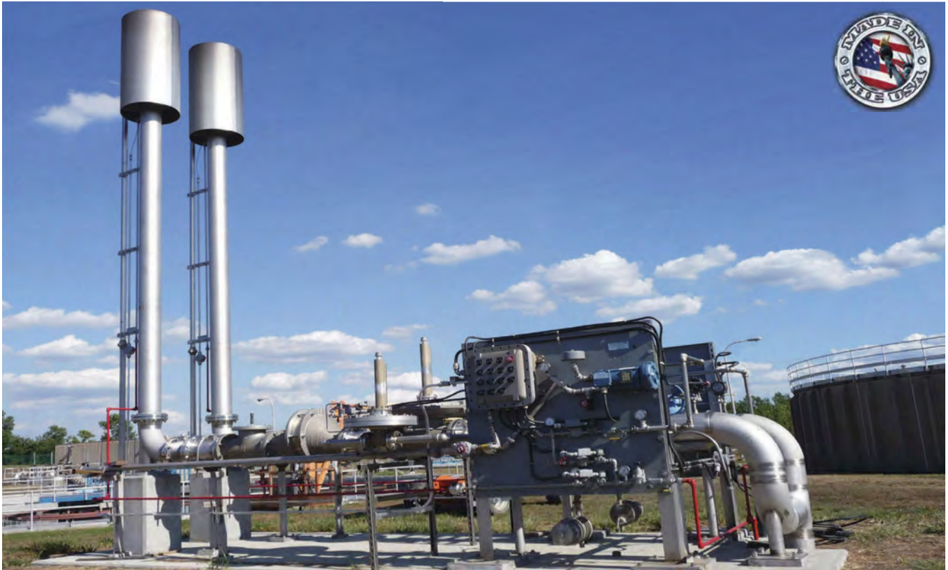
Ground Level Pilot Waste Gas System with two sets of Waste Gas Burners and Control Panels, Regulators & Flame Trap Assemblies
