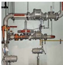
Regulator and Flame Trap Assembly
