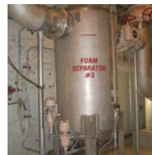
Foam Separator with High and Low Level Switches
