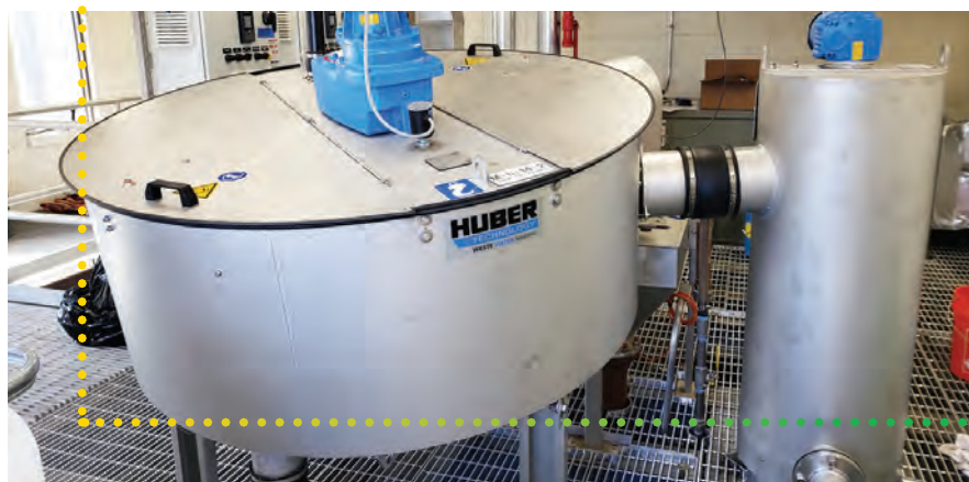
The Huber S-Disc thickener from Energetics, which provides 4% TS to the aerobic/anoxic digester.
