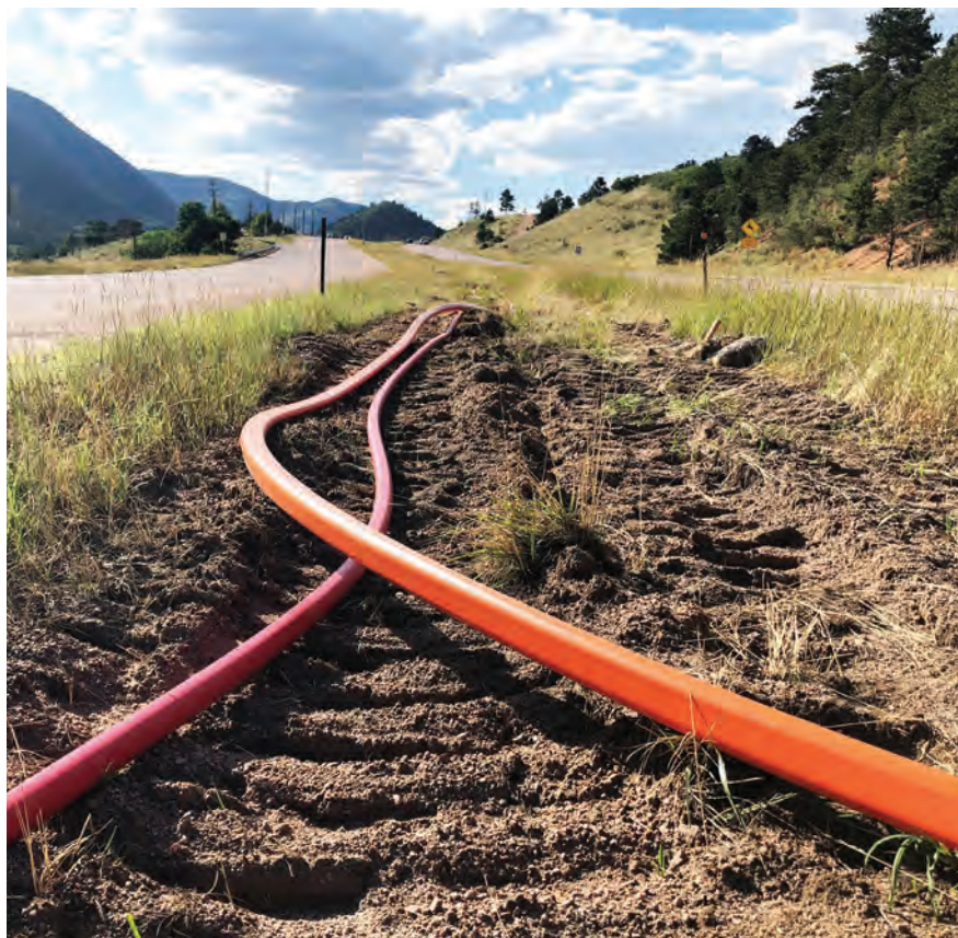
Photo demonstrates how public agencies should be dropping low-cost conduits into their water line jobs. (Photo: Dave Zelenok)
