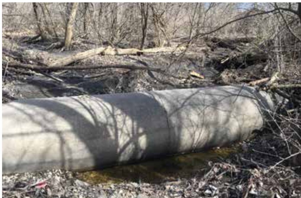
Exposed interceptor sewer pipe.
