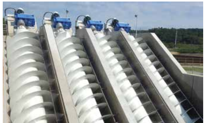
114-inch Open Screw Pumps in Roanoke, V.
