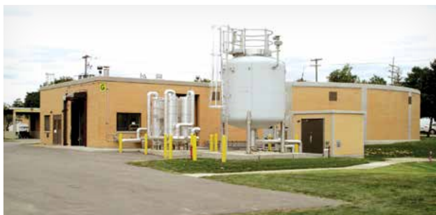
Figure 4. Digester gas treatment system
