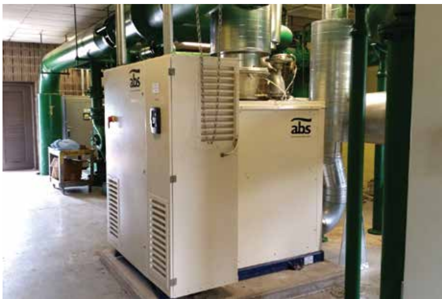
Figure 2. Aeration improvements, including blower and diffuser replacements
