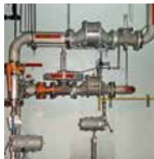
Regulator and Flame Trap Assembly
