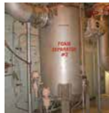
Foam Separator with High and Low Level Switches
