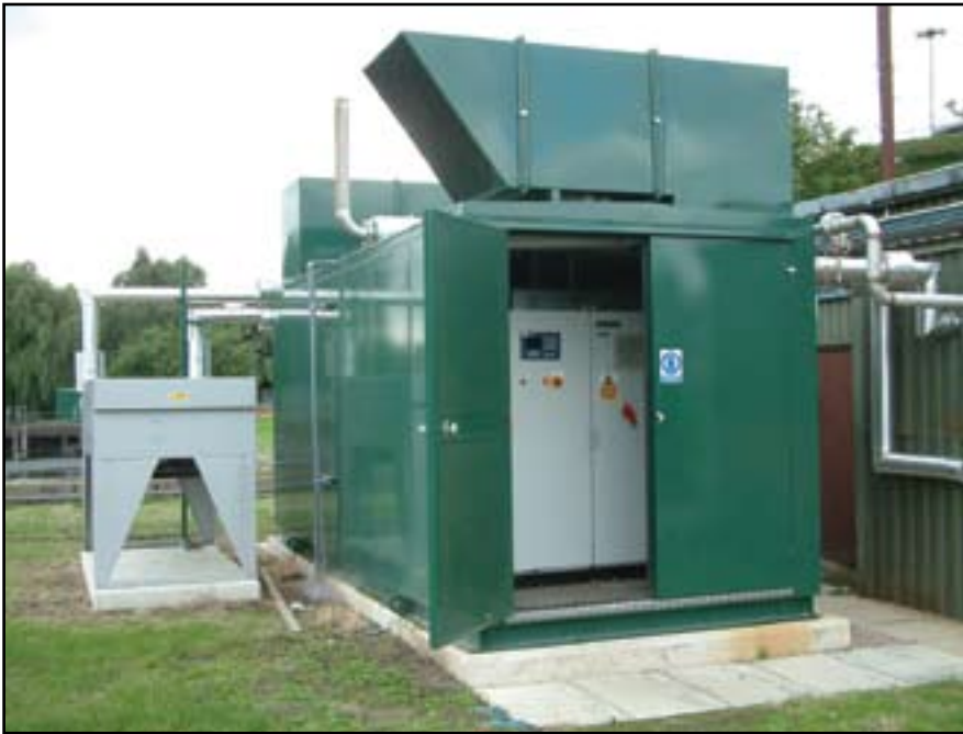
Typical 300KW CHP set installation (Courtesy Yorkshire Water).
