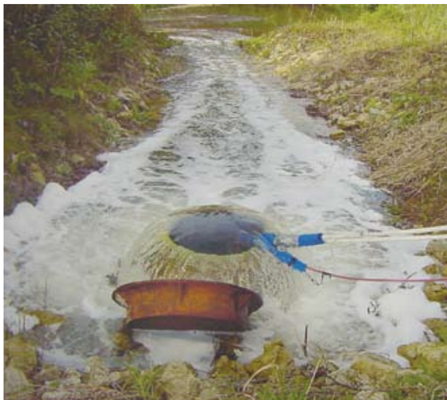
Temporary permitted overflow used to facilitate sewer rehabilitation.
