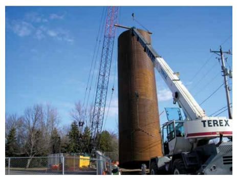
Initial support system being lowered into the 102' deep shaft for structure 83
