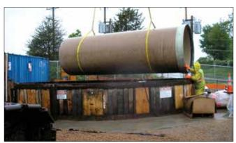
72" Diameter Hobas was used for the final carrier pipe
