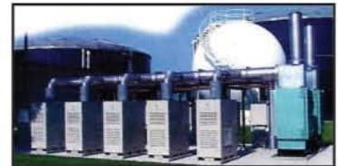
Utilize excess gas to produce electricity using Capstone microturbines with heat recovery.
