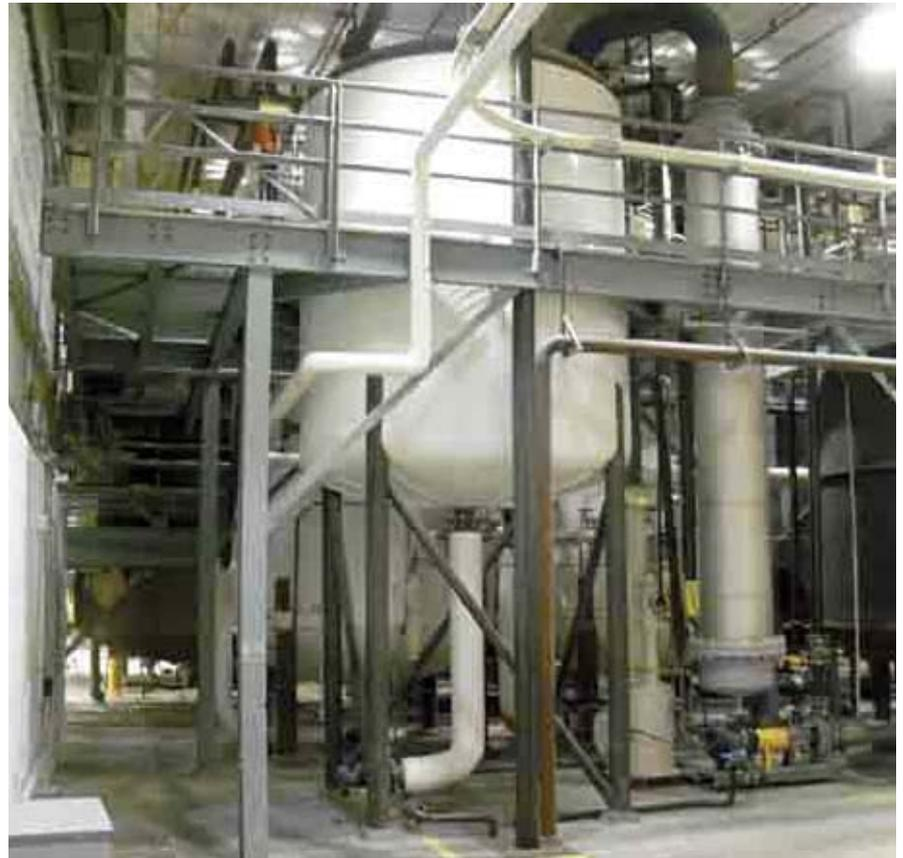
“Anaerobic digestion was a logical choice for treating the wastewater before it entered the publicly owned water treatment system.”
