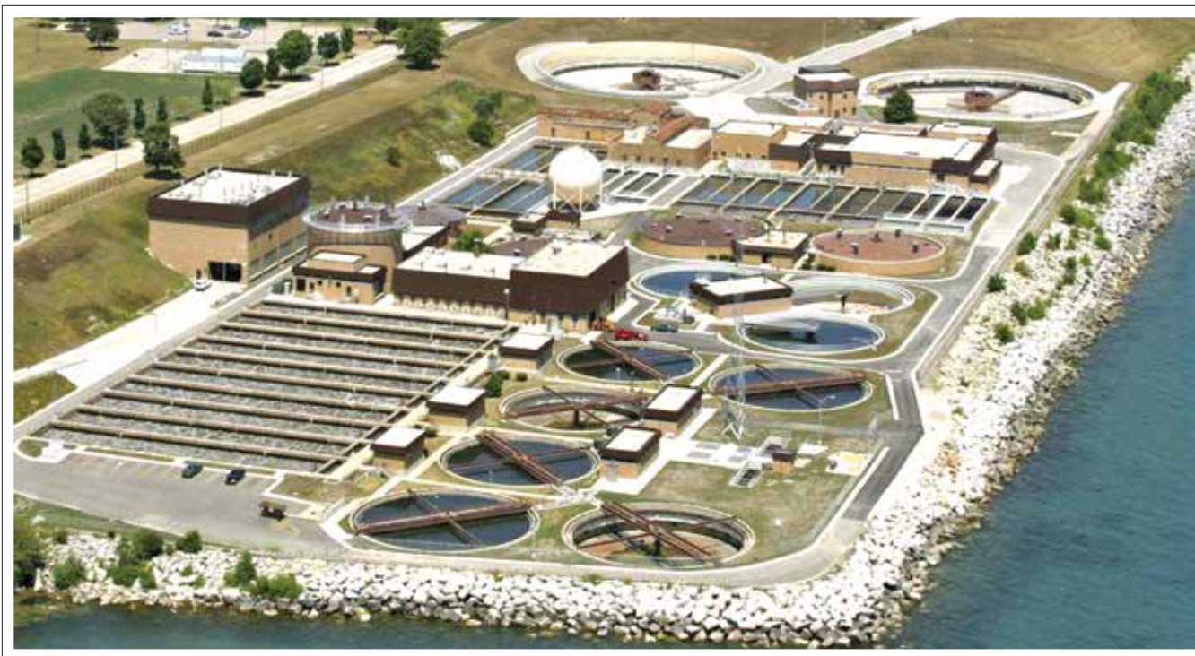
Present Day Aerial View of Racine Wastewater Treatment Plant
