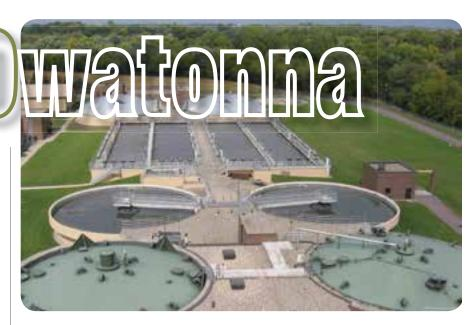
periodically cleaned by backwashing them with plant effluent to remove accumulated debris. Dual chlorine contact tank provides the proper detention for chlorine to kill harmful bacteria prior to discharging the effluent to the Straight River. Sulfur dioxide is added at the end of the tanks to eliminate the chlorine residual to further protect aquatic organisms.
