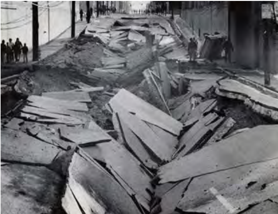
Louisville KY, sewer explosion, 1981
